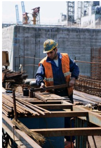
Workers at the steel framework base
