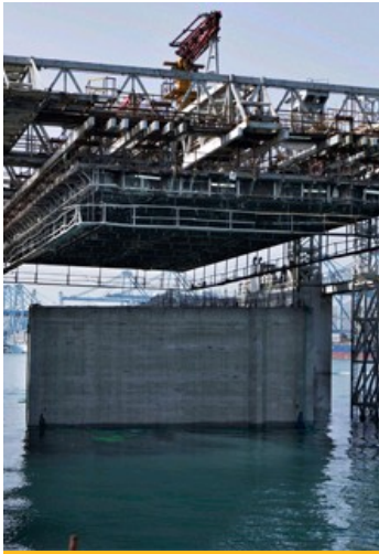
Coffer ready for launching
