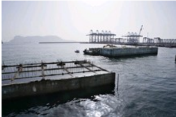
Manufactured coffers for pier construction.
