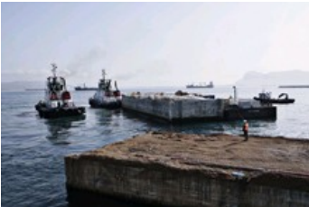
Transferring the coffer to its definitive location.
